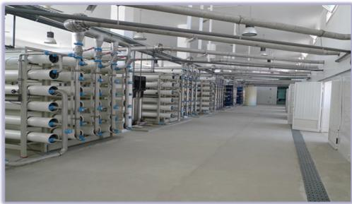
In an electricity driven process called electrolysis pure water can be split into its elements hydrogen  $H_2$  and oxygen  $O_2$ . If power from renewable resources is applied to the machine 100% green hydrogen is produced. However, electrolyzers must only be feed with pure water to avoid scaling and corrosion of inner cell parts. Even drinking water still contains too many minerals that would negatively disrupt the process.
